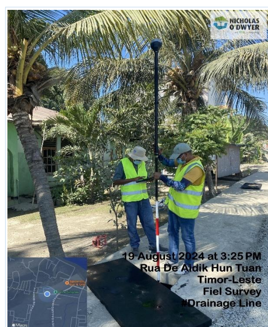
Figure 1: Nicholas O'Dwyer team of conducting a field survey for the drainage line in Rua de Aidik Hun Tuan
